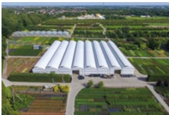
Nowy blok tunelowy. 2019 New tunnel block. 2019
